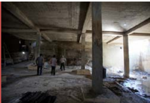
Construction inside the Kur reservoir
