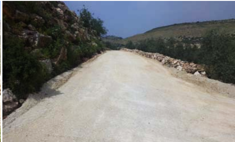
Road after rehabilitation
