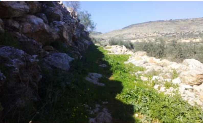
Road before rehabilitation
