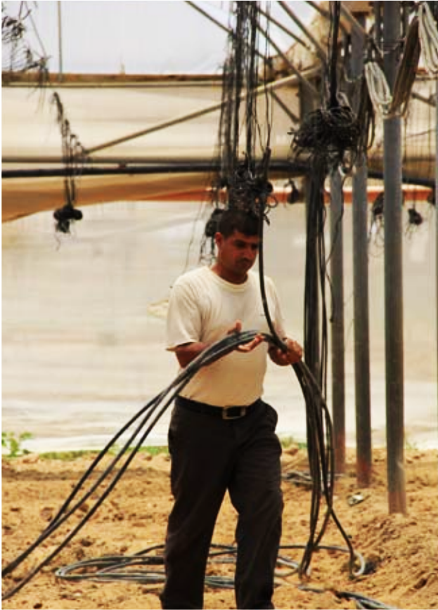
Basem Qudieh re-laying water irrigation lines in his greenhouse
