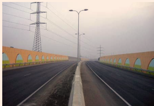
camouflaged walls along Israeli-only road 443
