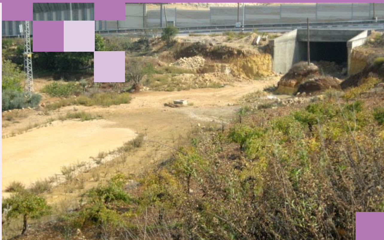
A tunnel that will serve as the only access point to the Husan and Battir villages under Israeli-only Road 375
