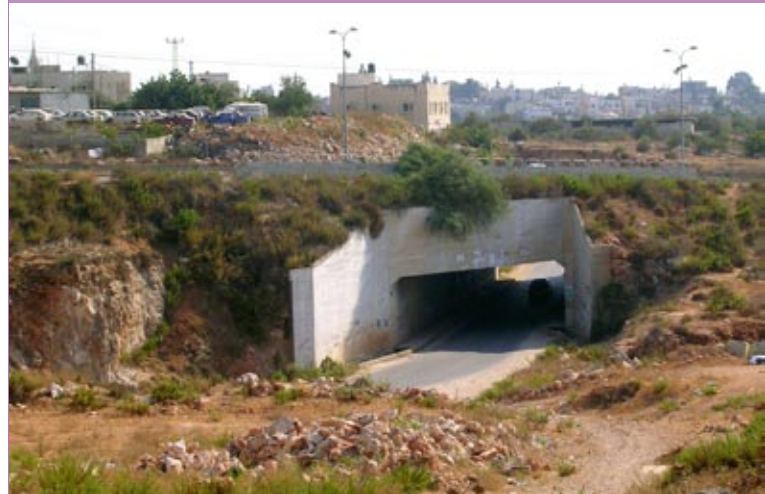
Tunnel leading to the Der Ballut sub-canton under Israeli-only Road 5
